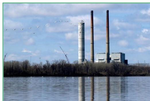
Both units at Sioux are equipped with wet flue gas desulfurization (FGD) equipment to comply with the Cross State Air Pollution Rule (CSAPR). CSAPR required significant reductions of sulfur dioxide (SO<sub>2</sub>) and nitrogen oxide (NO<sub>x</sub>) emissions on a regional scale by 2015. The FGD system at Sioux also provides significant co-benefits in complying with EPA's MATS rule for both mercury and particulate emissions.
