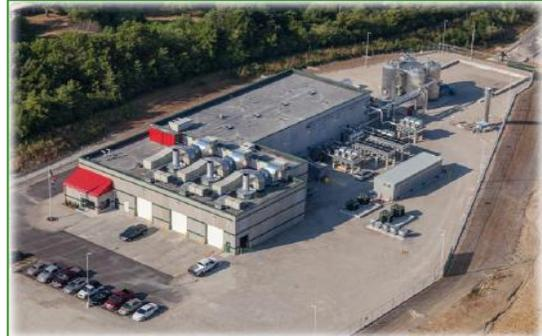
The MHREC began operation in June 2012. It has a total net summer capacity of 8 MW (net). This facility burns methane gas produced by the IESI Landfill in Maryland Heights, MO, in three Solar Mercury 50 gas turbines to produce electricity. The current contract with the landfill guarantees enough gas supply for three generators until 2022. In August 2012, the MHREC was certified as a qualified renewable energy resource by the MoDNR.
